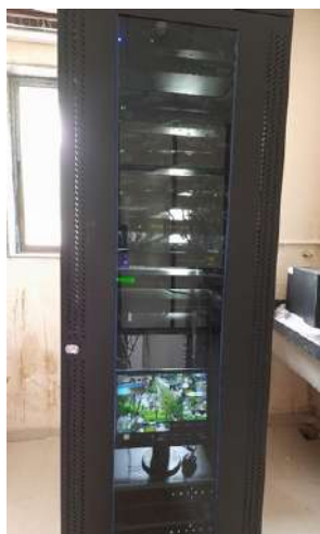
Server room rack with switches,Firewall
